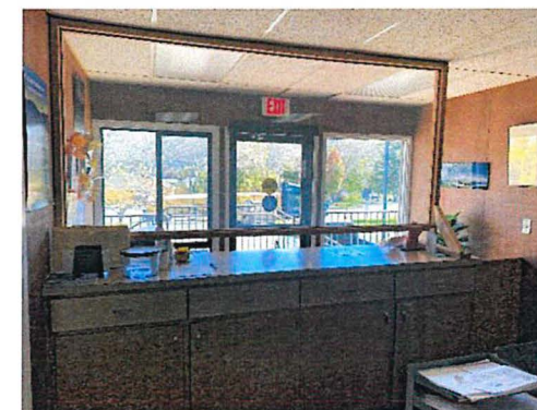
NEW WALL - DOOR - SECURITY TRANSACTION WINDOWS COUNTER - SNEEZE SHIELD TO BE REMOVED
