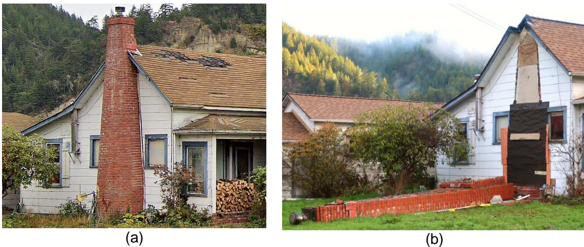
Figure 6.3. Example of masonry chimney collapse. (a) View before earthquake (undated Google maps street view image). (b) View after earthquake. Chimney fell away from home and now lying on its side in yard. It was fortunate that no adjacent structures were present that would have been impacted.
